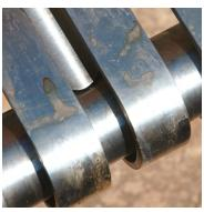
Stainless steel seat with discolouration due to weathering and non-maintenance.
