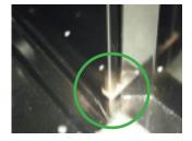
Spray copper grease generously onto/around latch mechanism and top and bottom hinges. The lower hinge area may be affected by dog urine, this should be wiped clean before applying copper grease.
